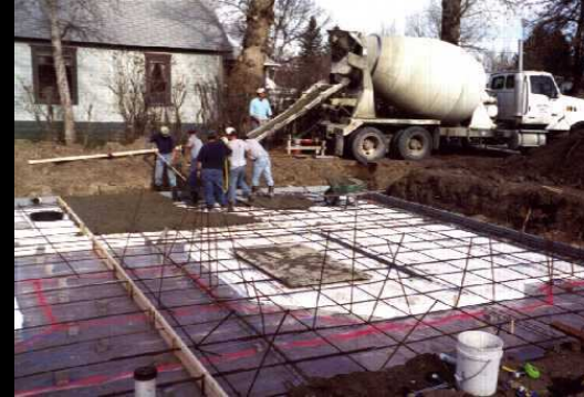
4" EPS Foam under crawl space floor.
