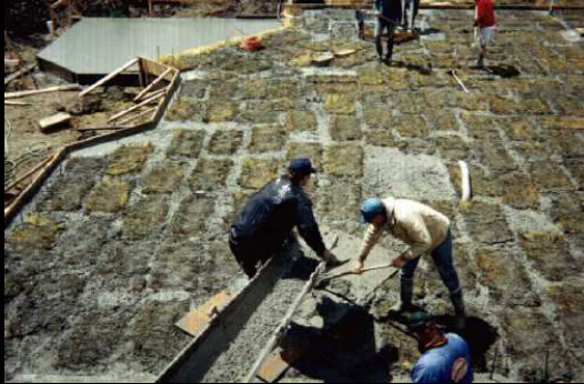
Bale Insulated Floor (don't do it!)
