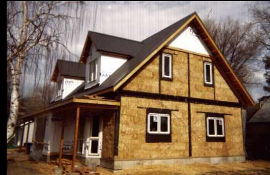
Straw Bale Walls
