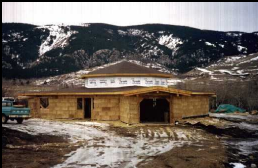
Straw Bale Walls
